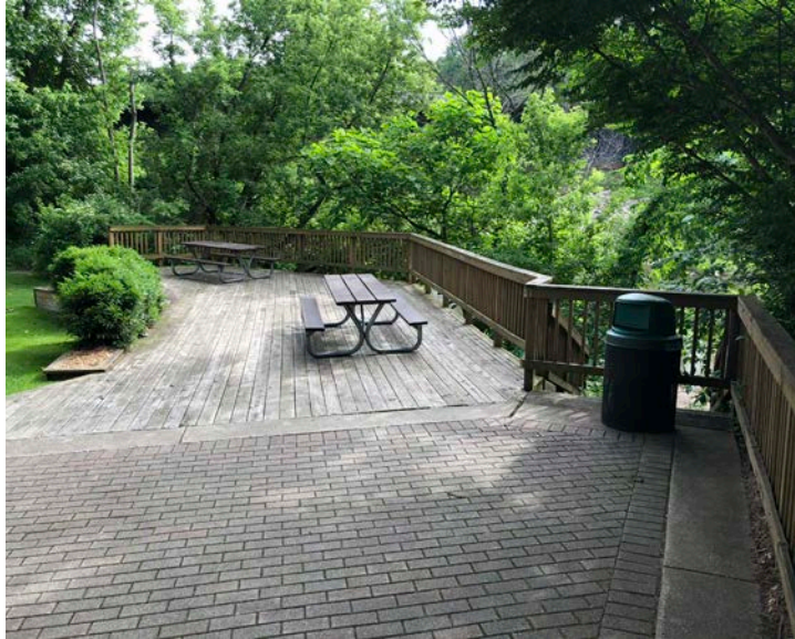
3 The existing bridge picnic area and overlook is in need of repair. Transitions between concrete, brick, and wood are abrupt and impair accessibility. Additionally, the handrails do not meet ADA standards. These facilities are highly used by visitors for picnics and photo opportunities.
