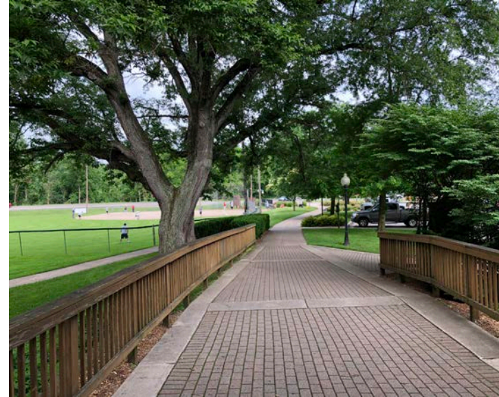
4 The centennial tree east of the Ada Covered Bridge should be protected and educational and interpretive signage should be provided. Railings along the covered bridge ramp are not ADA compliant. Additionally, settling of the sub-base has caused the pavers to become uneven.
