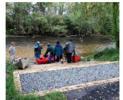
River Access Point with Improved Accessibility and Erosion Control
