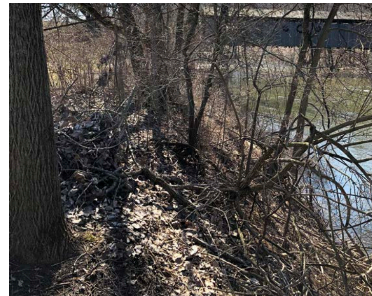
9 The riverbank exhibits erosion and is overgrown with invasive and non-contributor species that impede visual and physical access to the river. Riverbank improvements should include informal/low-impact opportunities for river access, stabilization, removal of invasive species, and planting of native species.
