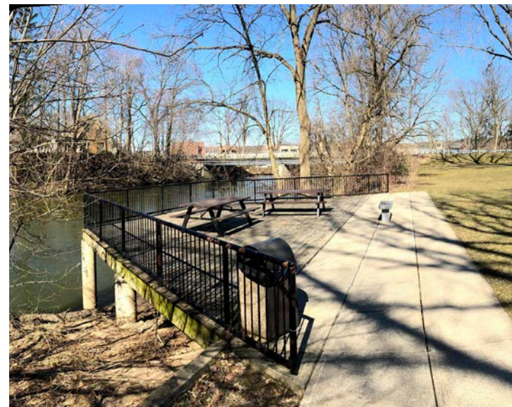
8 The river overlook deck requires updates for safety and accessibility compliance. In addition to daily use, the overlook deck also functions as a stage for the "Beers at the Bridge" summer concert series. Improvements should include universal accessibility features and interpretive/educational signage.
