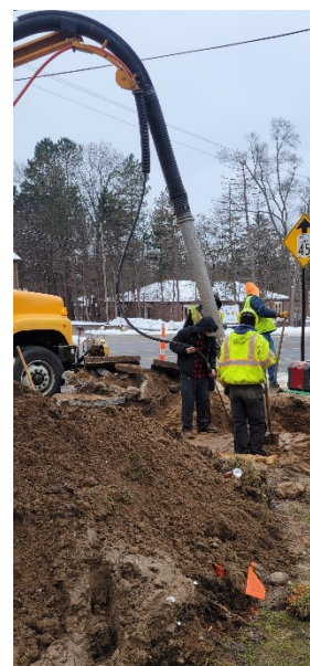
Excavation looking South West with above & underground electrical
