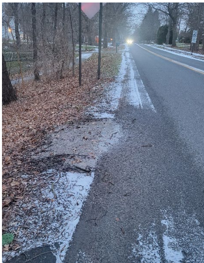
Sewage Overflow on South Side of Hall St
