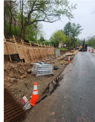
Soil Nail/Shotcrete Wall
