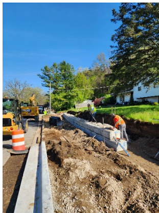
Segmental Block Wall
