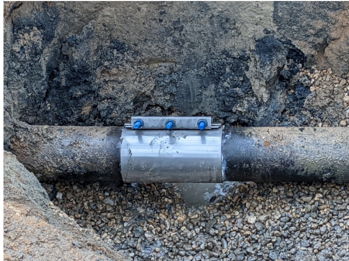
Completed Repair of 6" Force Main
