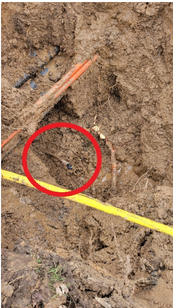
Cut water service between yellow gas line and orange fiber line and tree root.
