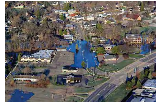
Figure I-3. The flood-prone area along Ada drive needs to be lifted about 3 feet to shed water.
