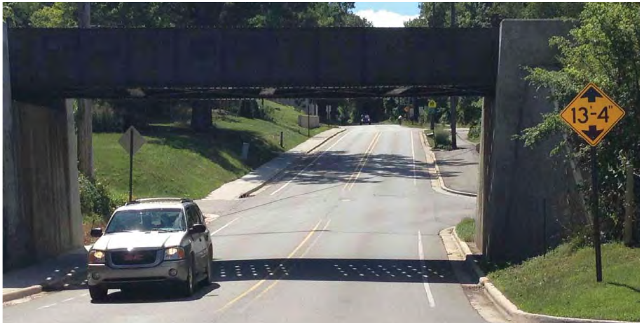
Figure IV-48. Wide lanes and shoulders on Ada Drive under the railroad tracks are an inducement to speeding. Figure IV-13.
