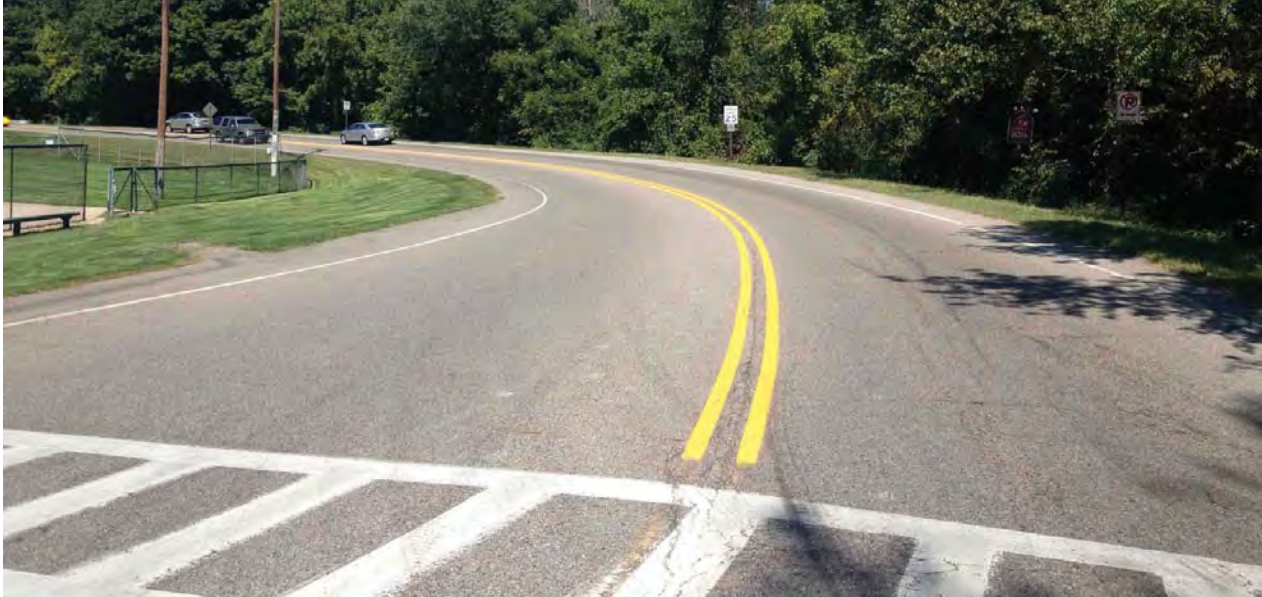
Figure IV-18. 12-foot lanes, shoulders, and no sidewalk make this stretch of Thornapple Drive particularly unsafe for walking.
