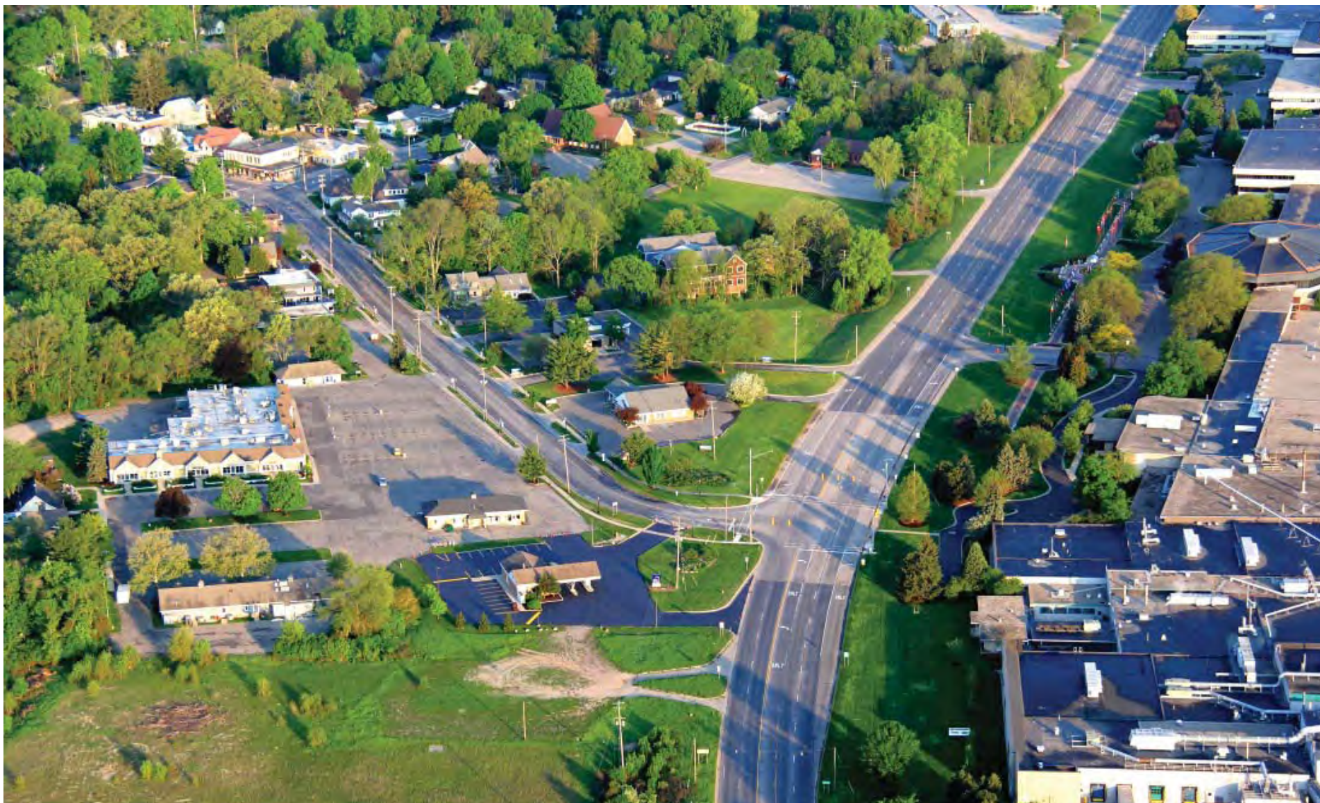
Figure I-11. Aerial view of M-21 and Ada Drive.
