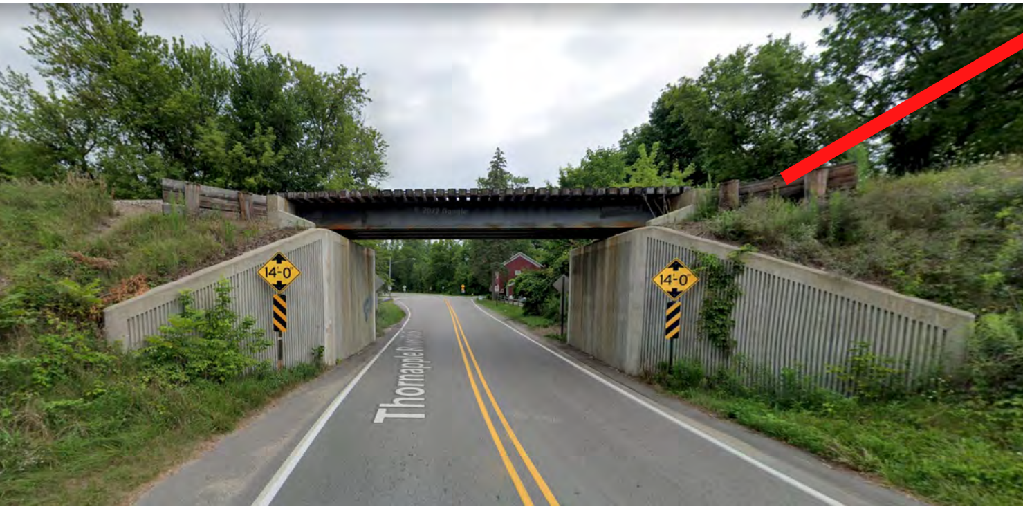
Thornapple River Drive NE rail tunnel
