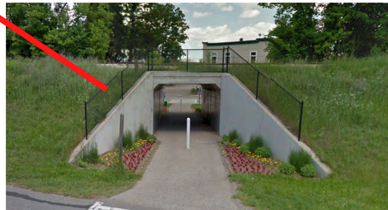
Ada Drive NE pedestrian tunnel
