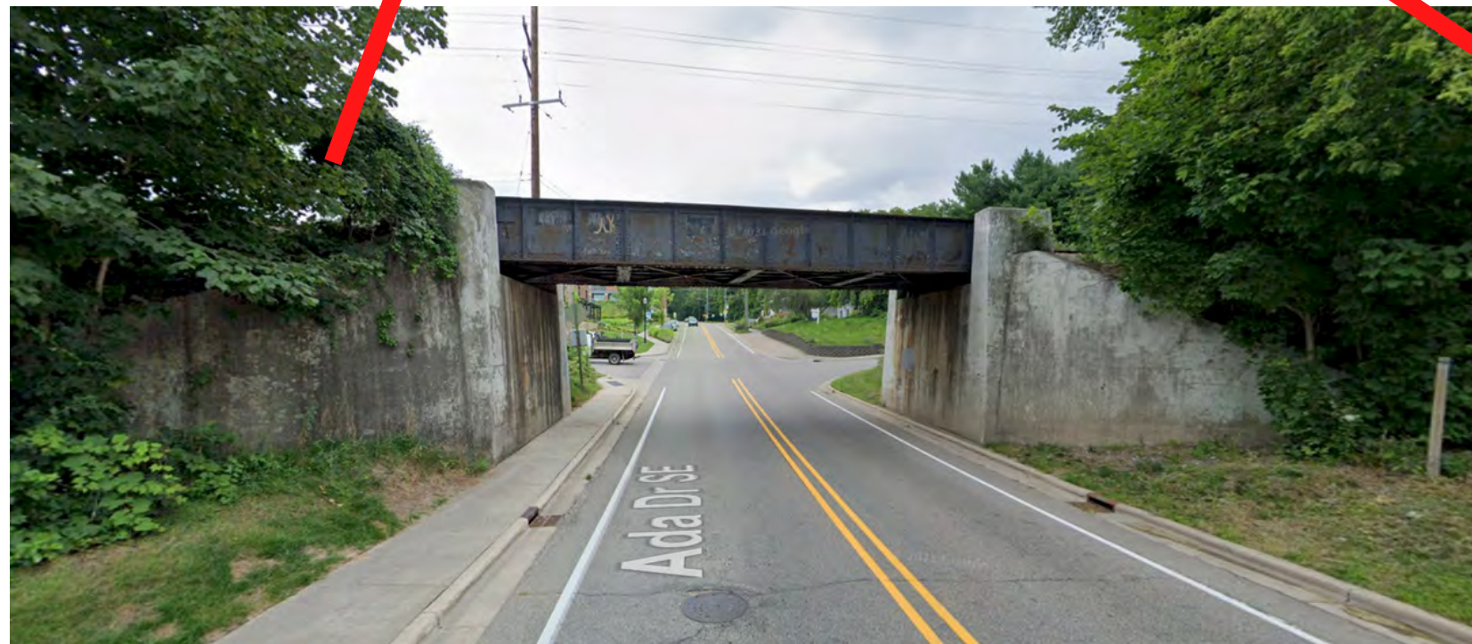
Ada Drive NE rail tunnel
